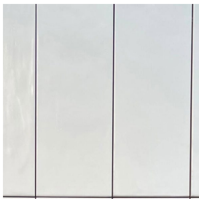
Wall tile Ceramic tile Colour: White Pattern: Vertical brickbond
